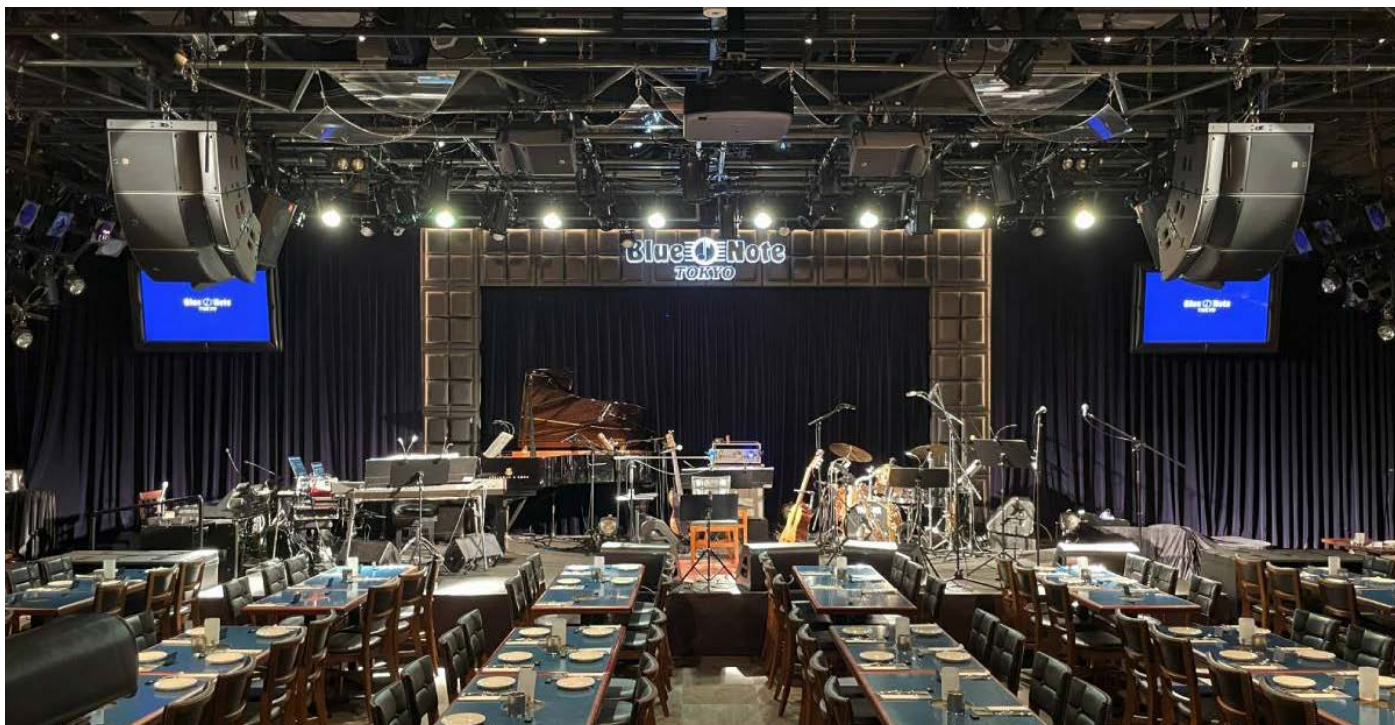
Blue Note Tokyo main L/R installation of two hangs of one L-Acoustics A15 Focus and two A15 Wide per side.
