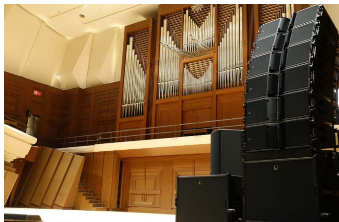
L-Acoustics Kara II atop two SB18 subwoofers. One L-Acoustics X12 per side provide in-fill.
