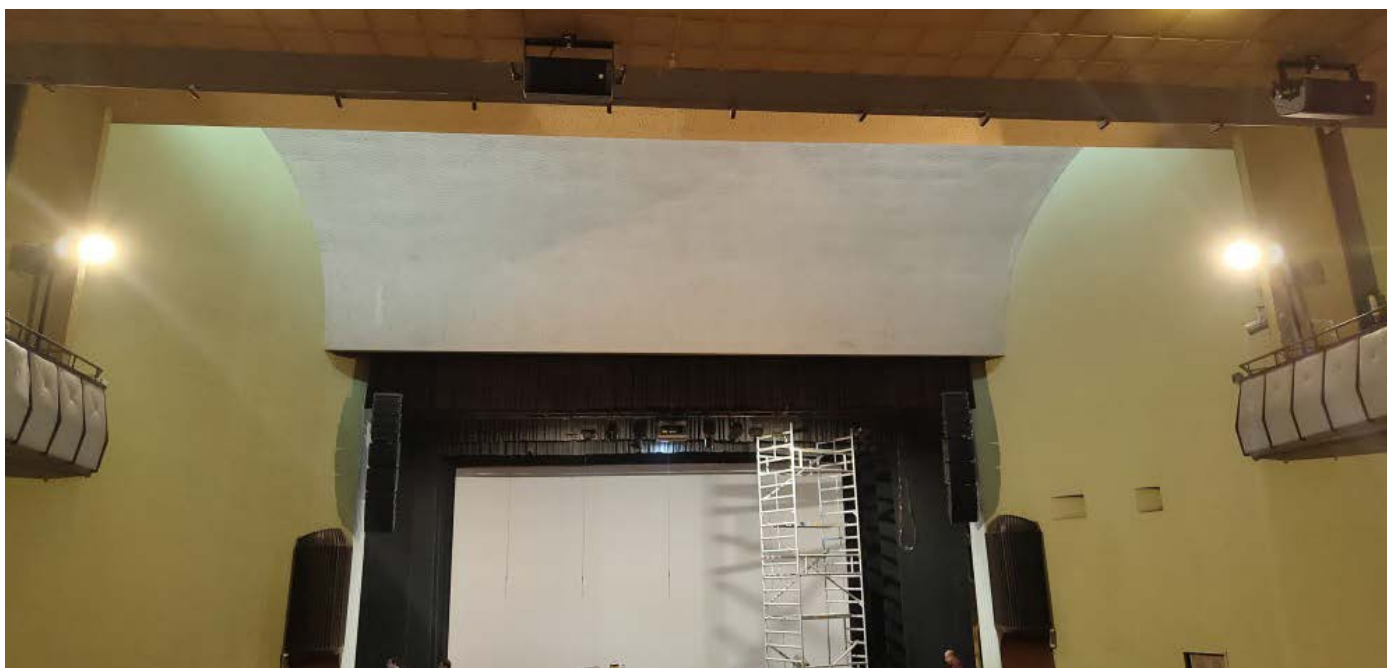
4 units of the HOPS5 as delays under the balcony and 2 units of the HOPS5 as balcony delays.
