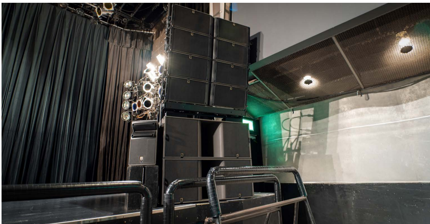
Spotify O-WEST's main left-right system of four L-Acoustics K2 stacked atop two KS28 subwoofers with in-fill delivered by A10 Wide speakers in Shibuya, Tokyo.
