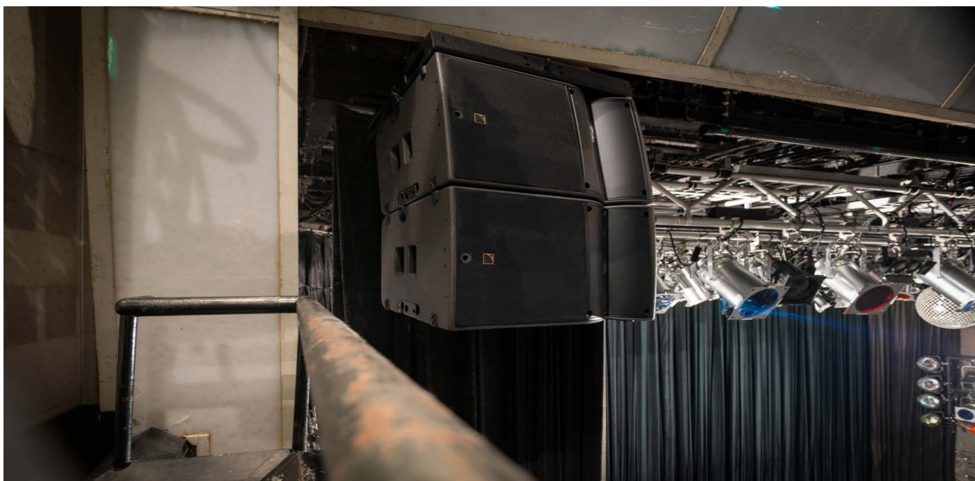
Above each main left-right stack in Tokyo's Spotify O-WEST venue are two L-Acoustics A15 Focus covering audiences on the second-floor.
