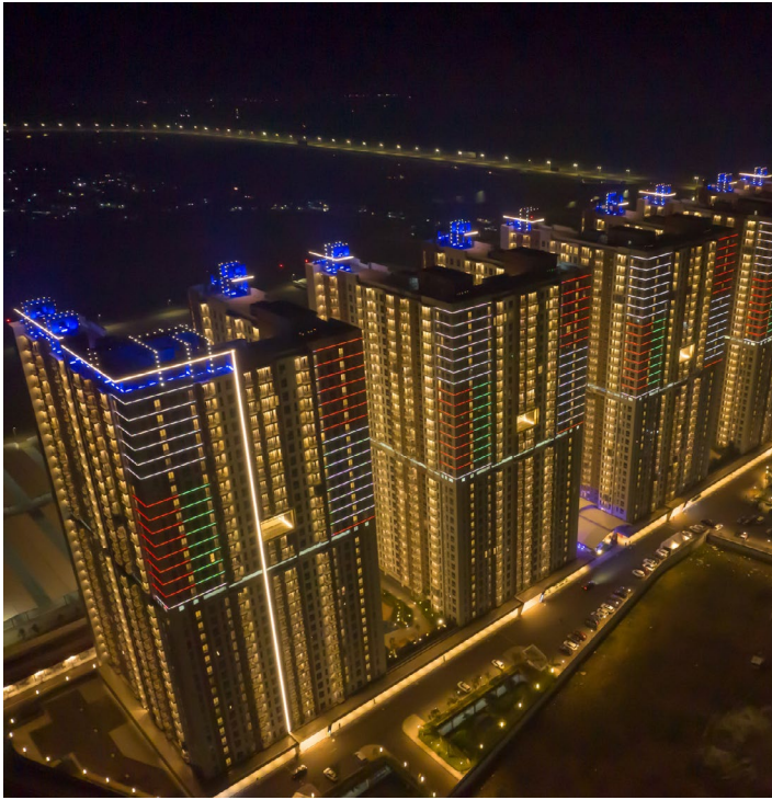
Harman Professional Solutions illuminated the new Tokyo Riverside Apartments with Martin VC-Dot 1 outdoor LED lights
