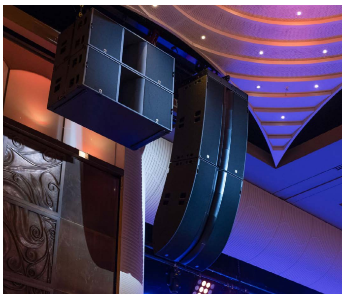
Encore Event Technologies designed a professional sound system of an L2/L2D pair with a companion pair of L-Acoustics KS28 subwoofers in the Crown Palladium Ballroom.
