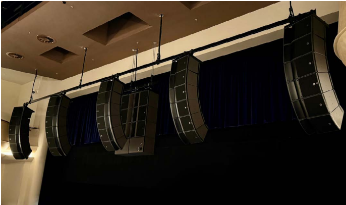
The L-ISA configuration at Ho Bee Auditorium features five hangs of five L-Acoustics A15i Focus and one A15i Wide each, with eight L-Acoustics KS21i centre-hung subwoofers.
