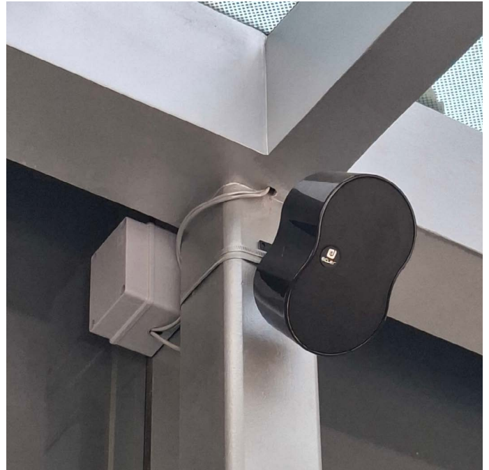
Special ties were used to fasten the speakers.
