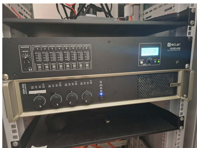
The Ecler VID-24Q digital 4-channel DSP amplifier and the HUB1408.
